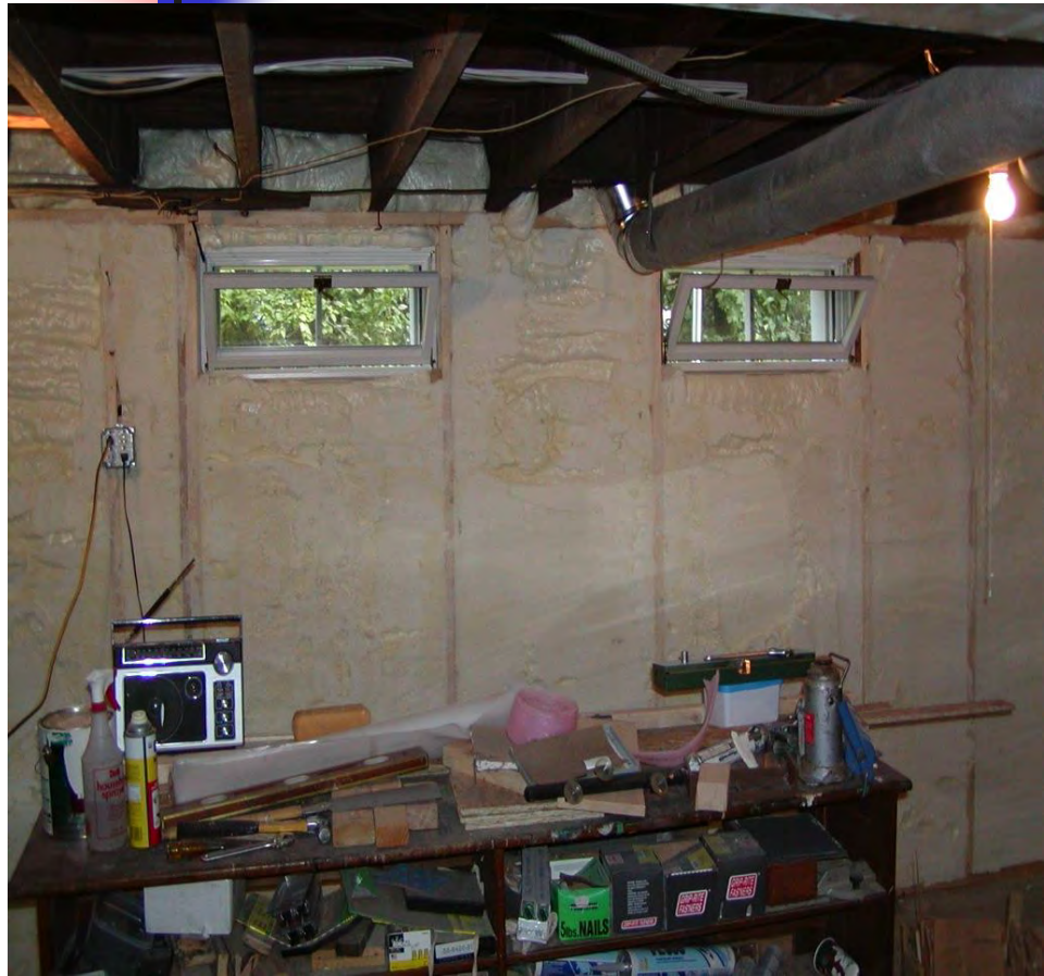
Open-cell in basement
